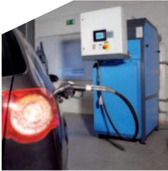
Natural gas fuel station
